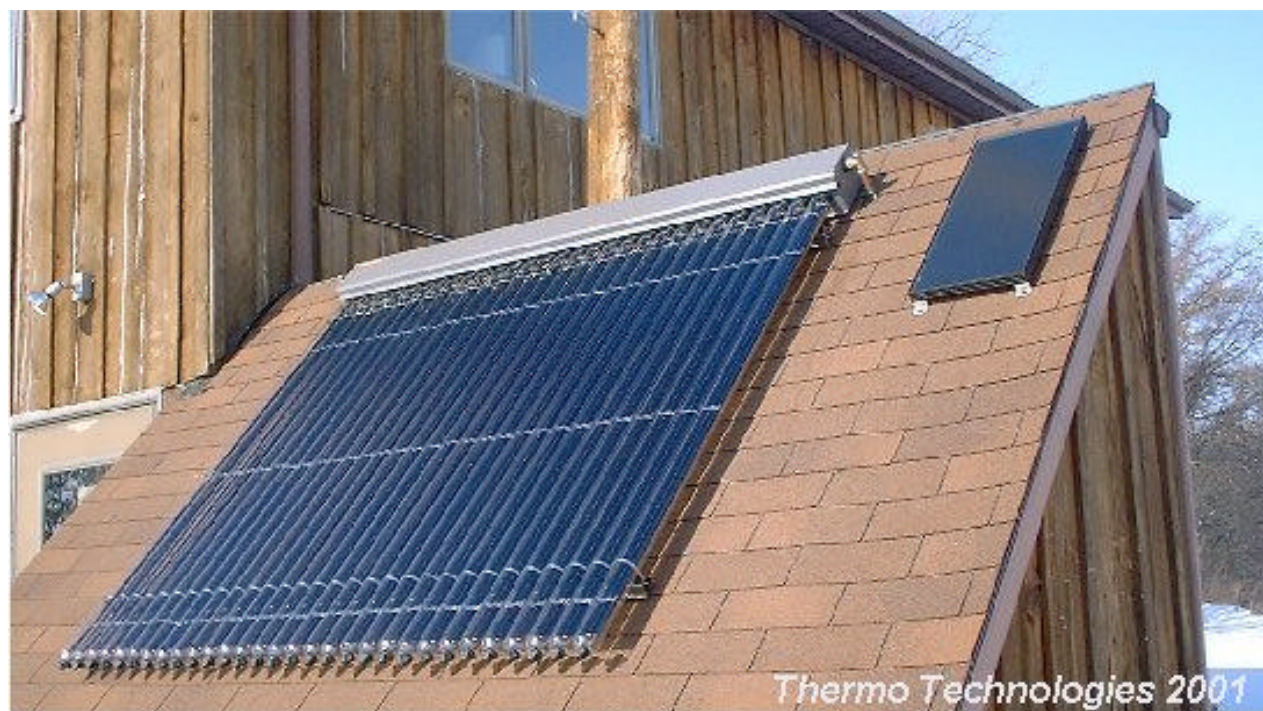
Figure 10. A solar water heater with a PV panel that powers the circulation pump.
