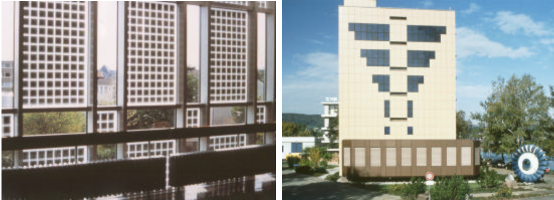
Figure 2. Left: Crystalline silicon PV cells between glass panes in a German building (Pilkington Solar AG). Right: PV modules as a patchwork on a building in Switzerland (Solution AG).
